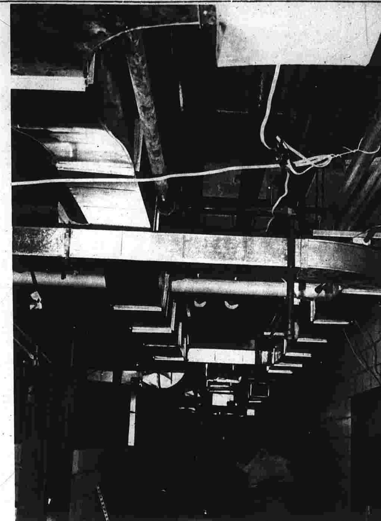
A basement corridor in the wing shows the many pipes and ducts that the ceiling will conceal.
